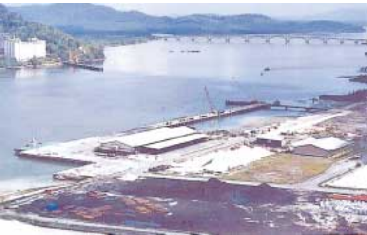
Lumut Maritime Terminal (LMT).
