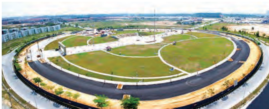
Bulatan 18, Public Park in construction phase
